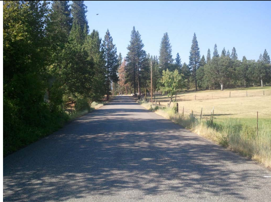
Figure A-3 Section 1, Location 3. Road width is 22 feet, with east and west shoulder widths of 2 feet and 1 foot, respectively. Grade is 1.2%.
