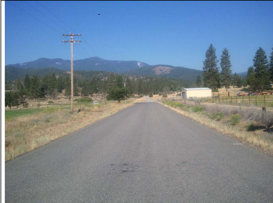
Figure A-1 Section 1, Location 1. Road width is 24 feet, with east and west shoulder widths of 1 and 3 feet, respectively. Grade is 2.5%.
