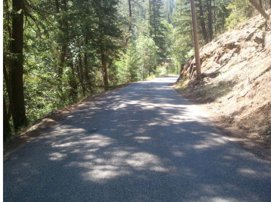
Figure A-15 Section 4, Location 1. Road width is 11.5 feet, with east and west shoulder widths of 1 foot. Grade is 1.8%.
