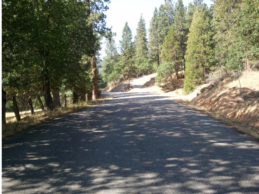
Figure A-9 Section 3, Location 3. Road width is 22 feet, with east and west shoulder widths of 3 feet and 1 foot, respectively. Grade is 1.3%.
