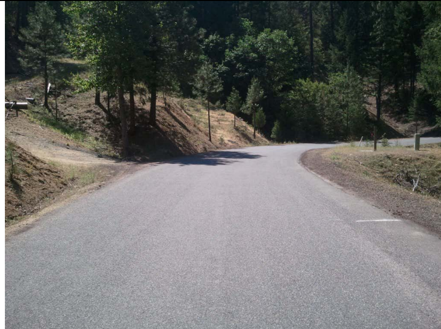
Figure A-17 Section 5, Location 1. Road width is 19 feet, with east and west shoulder widths of 1 and 4 feet, respectively. Grade is 2.4%.
