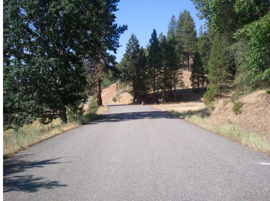
Figure A-7 Section 3, Location 1. Road width is 23 feet, with east and west shoulder widths of 2 feet and 1 foot, respectively. Grade is 1.3%.
