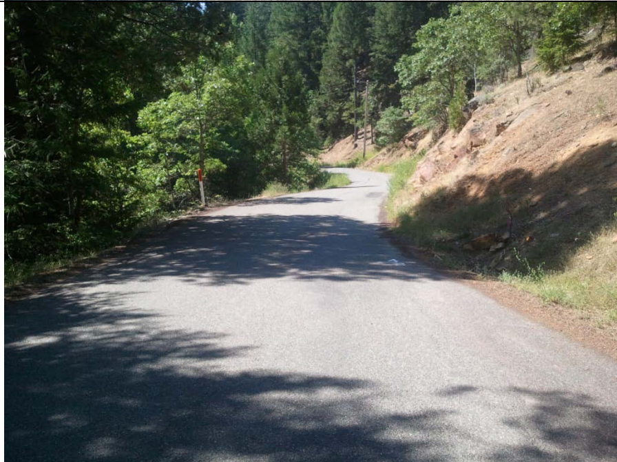
Figure A-14 Section 4, Location 0. Road width is 21.5 feet, with east and west shoulder widths of 2 feet and 1 foot, respectively. Grade is 1.1%.
