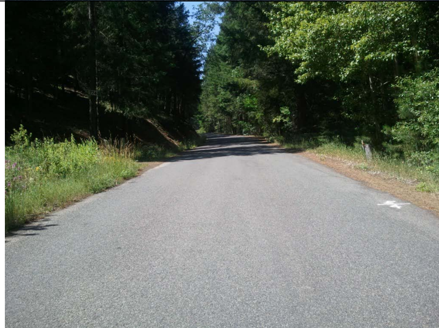
Figure A-16 Section 5, Location 0. Road width is 21 feet, with east and west shoulder widths of 1 foot and 3 feet, respectively. Grade is 3.5%.
