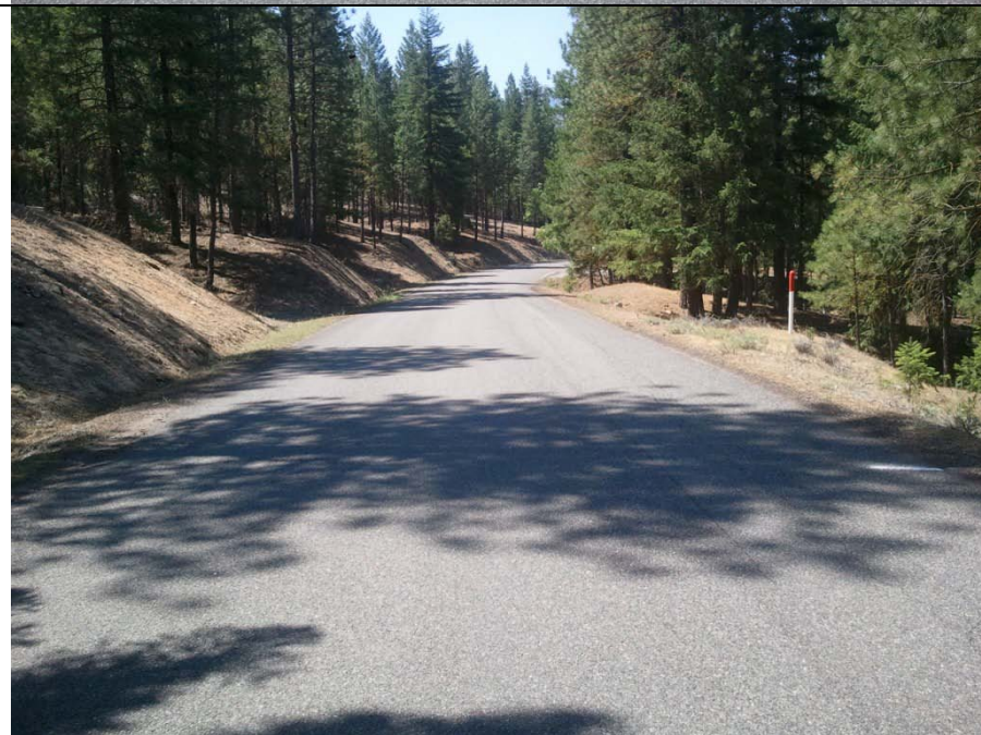
Figure A-18 Section 5, Location 2. Road width is 22 feet, with east and west shoulder widths of 1 foot and 3 feet, respectively. Grade is 1.8%.
