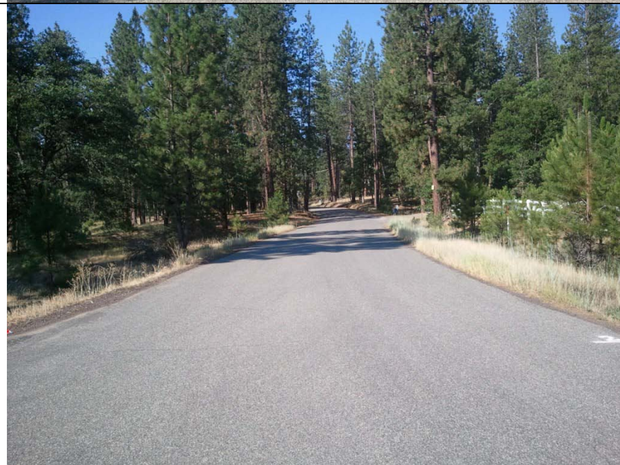
Figure A-4 Section 2, Location 0. Road width is 25 feet, with east and west shoulder widths of 3 and 2 feet, respectively. Grade is 2.9%.
