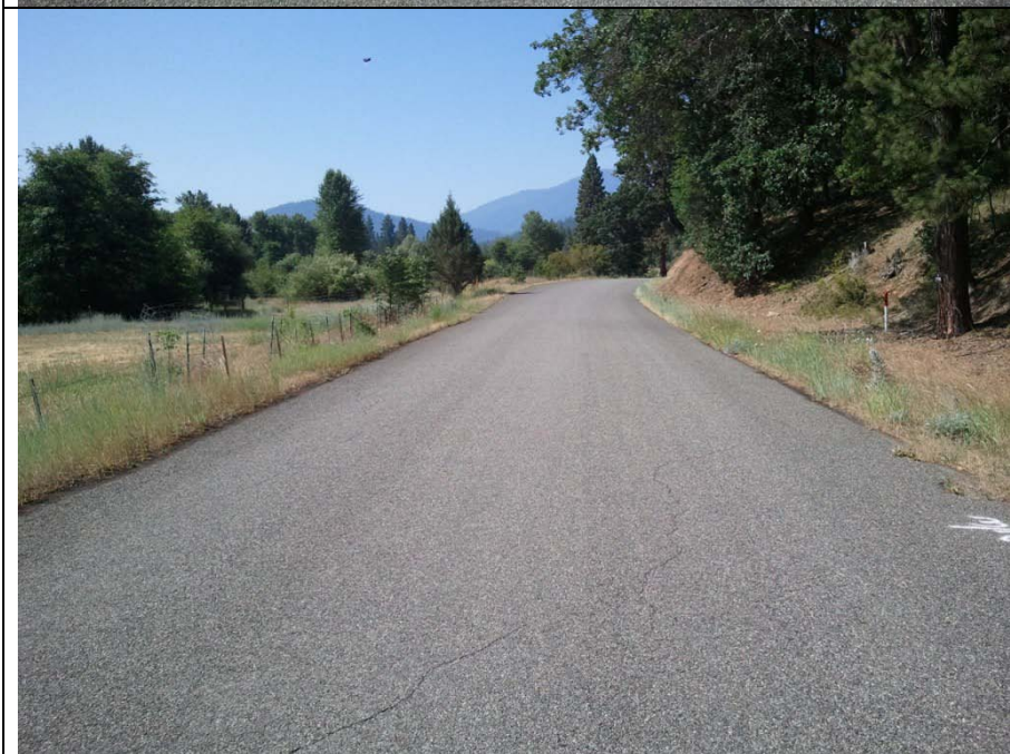
Figure A-6 Section 3, Location 0. Road width is 22 feet, with east and west shoulder widths of 2 and 3 feet, respectively. Grade is 1.8%.
