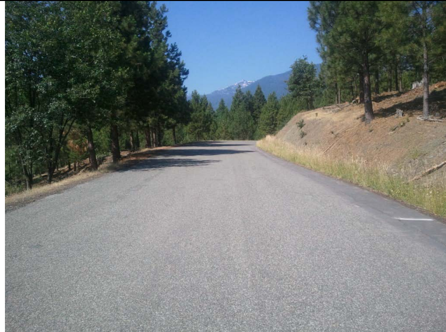
Figure A-11 Section 3, Location 5. Road width is 25 feet, with east and west shoulder widths of 3 feet and 2 feet, respectively. Grade is 2.7%.
