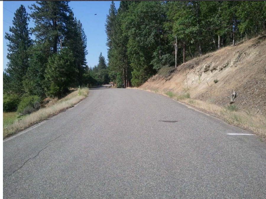
Figure A-8 Section 3, Location 2. Road width is 23 feet, with east and west shoulder widths of 2 and 7 feet, respectively. Grade is 4.5%.
