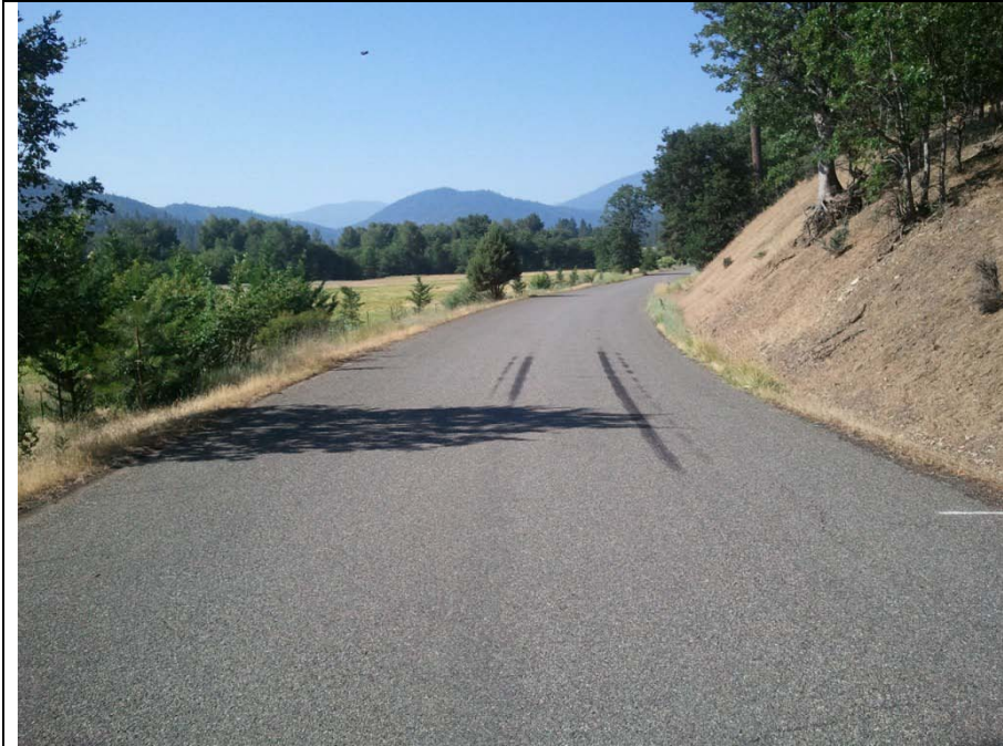
Figure A-5 Section 2, Location 1. Road width is 22 feet, with east and west shoulder widths of 3 feet and 1 foot, respectively. Grade is 0.6%.
