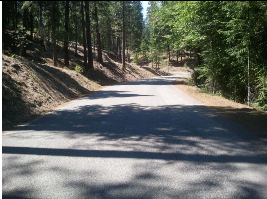
Figure A-20 Section 6, Location 1. Road width is 19.5 feet, with east and west shoulder widths of 1 foot and 4 feet, respectively. Grade is 3.7%.
