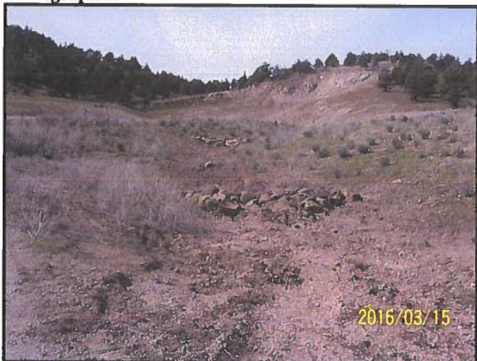
View of erosion control measures completed on the swale.
