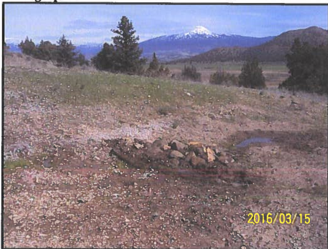
One of 3 rock dissipaters constructed to control erosion
