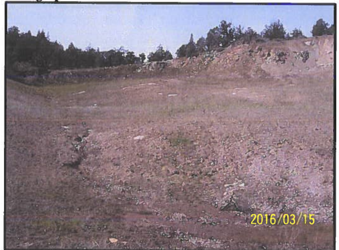
Phase 1 of the quarry as viewed from the pad site.
