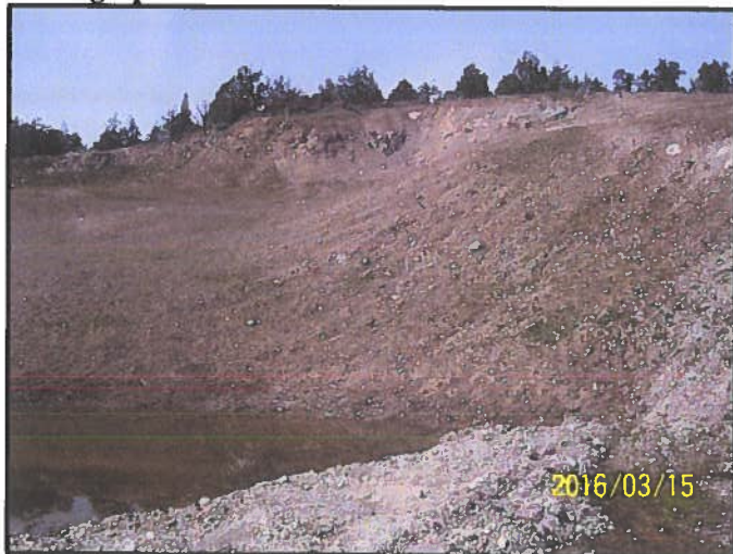
Over steepened area located at the top center of the cut face.
