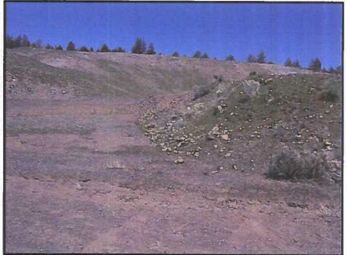
View of the toe of the slope below the processing area.
